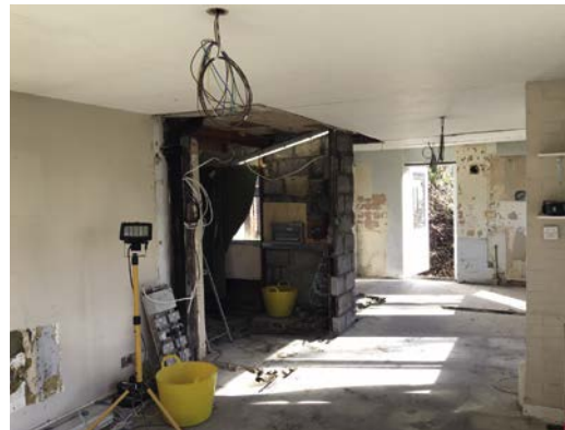
Good progress being made at the new bungalow.
